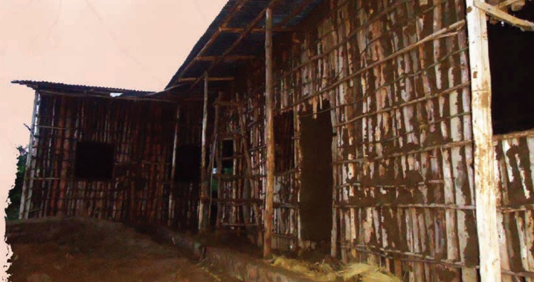
It's almost finished. The inside will have concrete flooring, and the outside still requires a fair amount of work. The outside walls will be covered with a cement mix. The first two rooms are designated to accommodate guests.
